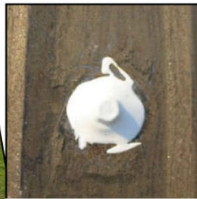
Each fastener receives a generous dollop of Rivet Guard™ to lock out moisture.
