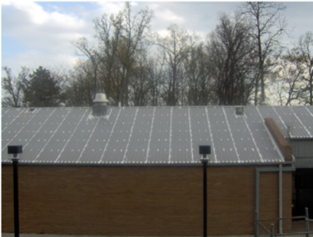
All seams & fasteners sealed
