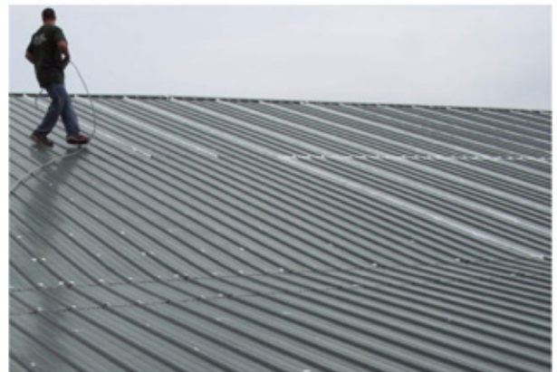
Step 7: Seal Seams with RivetGuard
