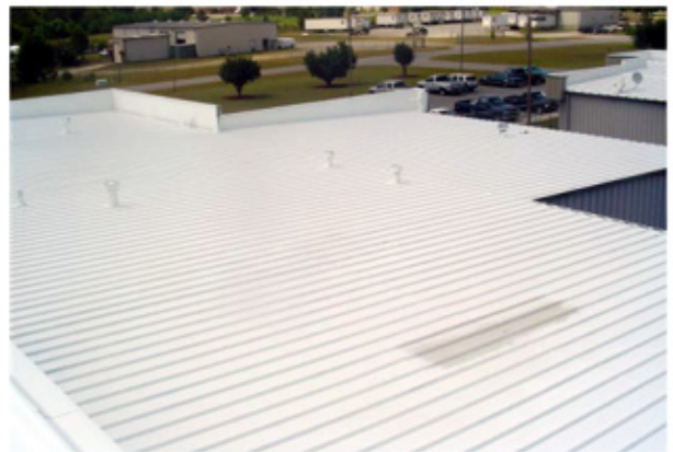
Step 10: Completed Roof
