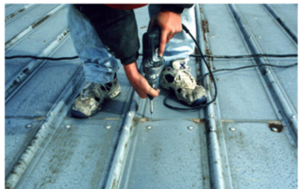
Install Additional Fasteners as Needed
